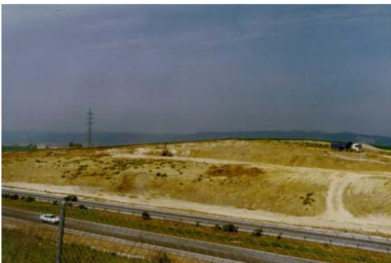
Figure 1. Sliding embankment of the CN-IV in P.K. 385.750
