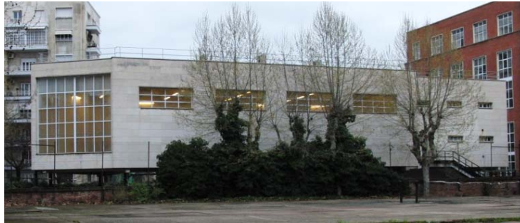
Figure 1. External photograph of the structure
