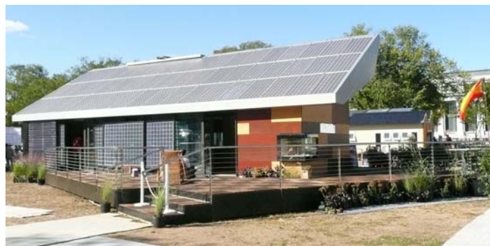
Fig.4 “Photograph of the south façade at UPM”
