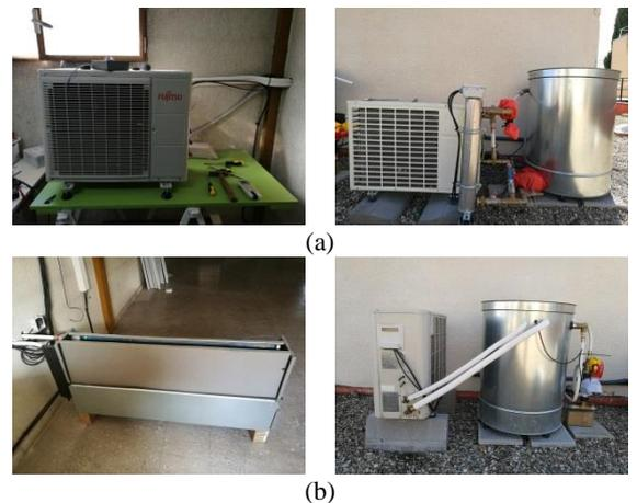
**Figure 3:** Images of the PV heat pump prototype installed in Madrid (Spain), composed of the tested system (a) and the auxiliary system (b).
