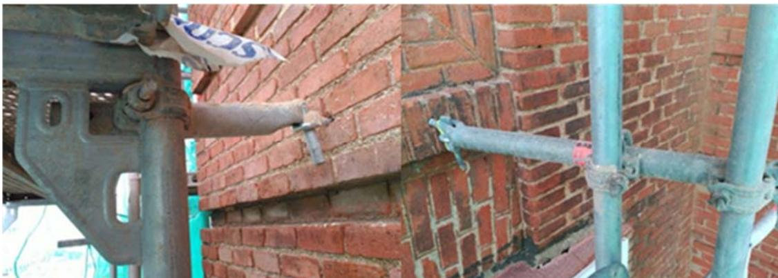
**Fig. 1: Different solutions for fastening façade using plugs.**
