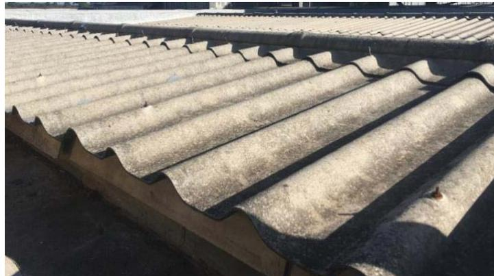
**Fig. 1: Fiber cement cover currently in use**
