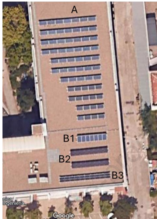
Figure 1 Google Maps view of the PV plant.
