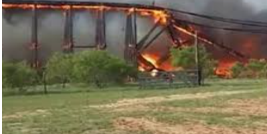
Figure 2.9: Texas wooden trestle railroad bridge fire
