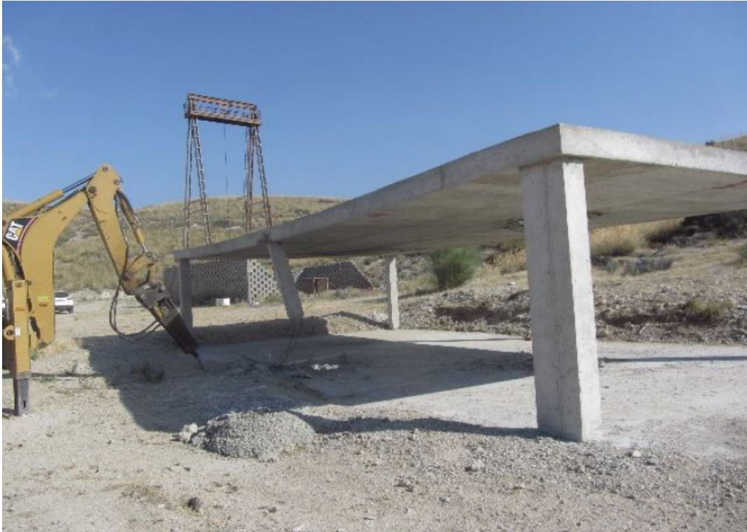
Figure 2.30: Two-span structure: demolition of central column using a pneumatic hammer.
