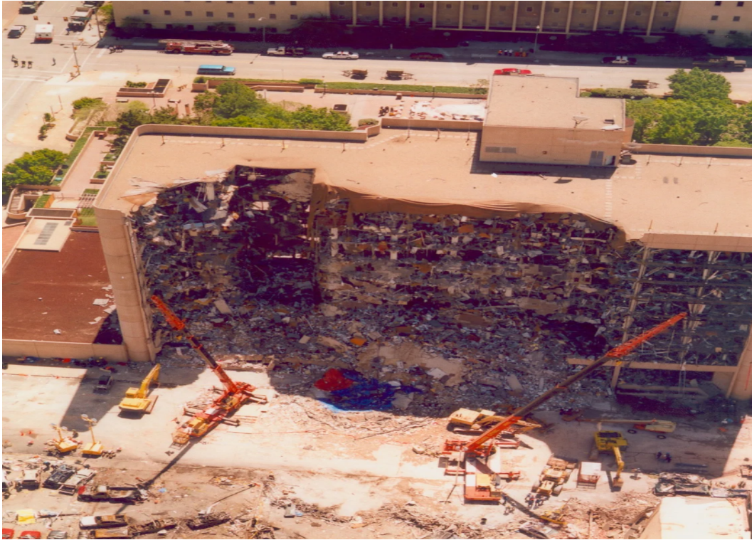
Figure 2.5: Alfred P. Murrah Federal Building in Oklahoma City on April 19, 1995
