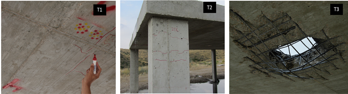
Figure 4.24: Damage to concrete after each test.
