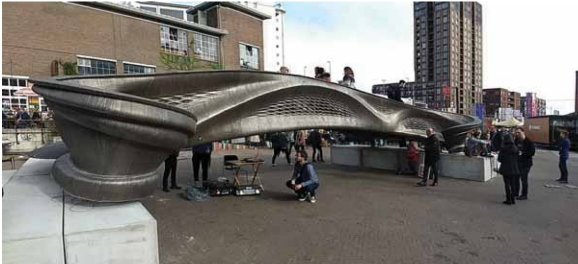
Figure 71. 3D printed bridge.MX3D. 2021.
