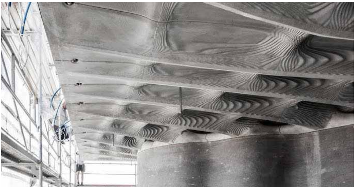
Figure 110. 3D printed concrete slab DFAB House. DBT. 2018.
