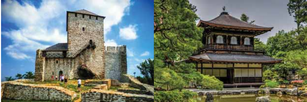
Figure 58 (Left). Western stone building. Figure 59 (Right). Eastern wood building.
