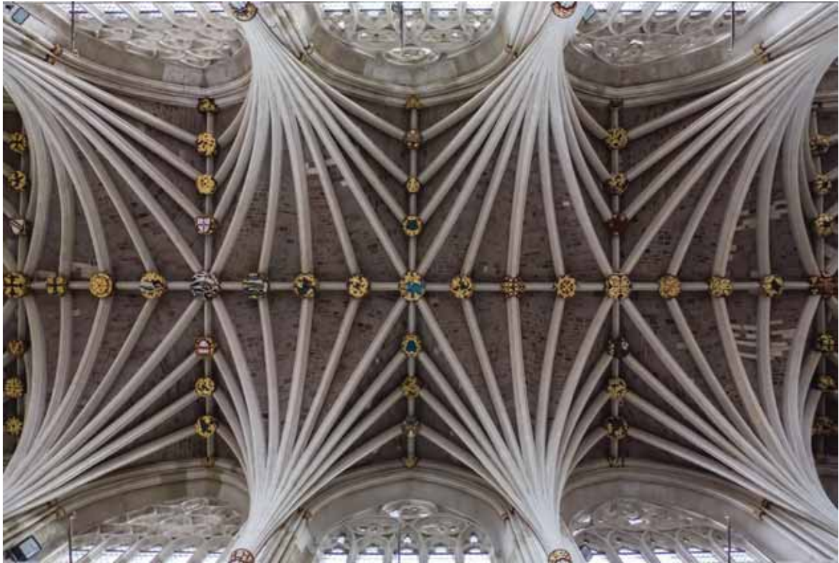
Figure 1. Exeter Cathedral. Example of a decorated structural stone vault. 1440 a.c. Exeter, United Kingdom.
