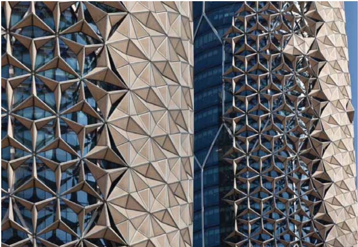
Figure 111. Parametric façade Al-Bahar Tower.AEDAS. 2012.
