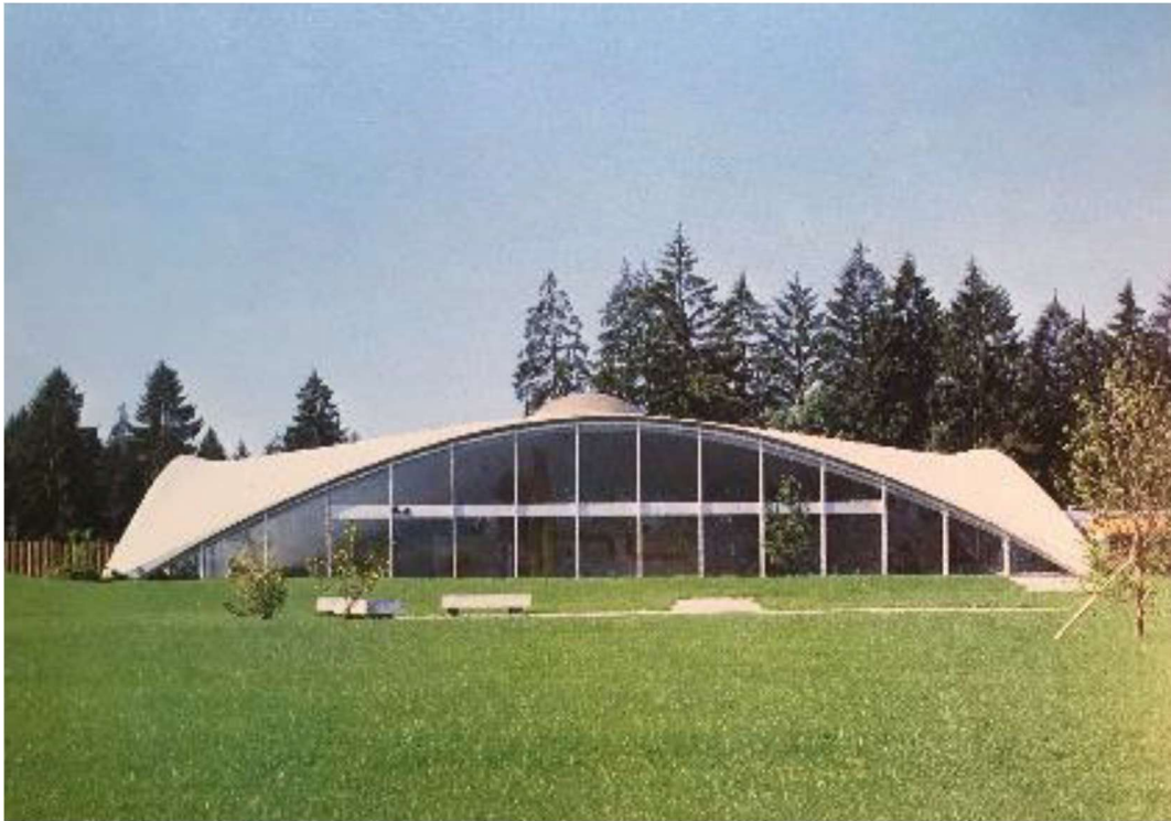
Fig. 26. Vista exterior. Heimberg swimming pool
