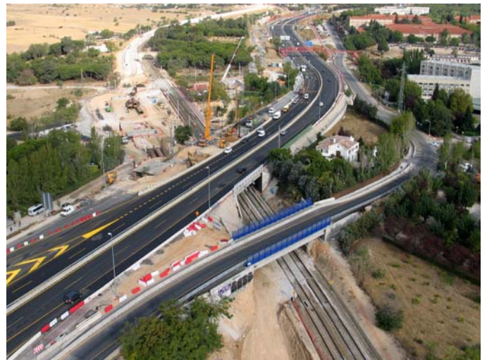
Figure nº 3 The new bridge E-2 and to the bridge E-3A/3B in construction
