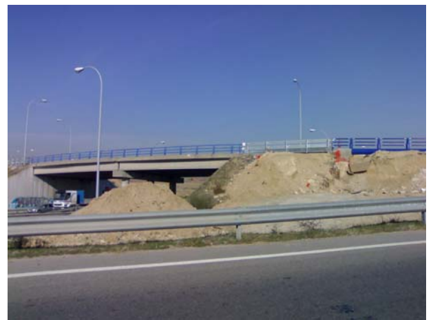
Figure 2. Central and lateral bridges prior the construction
