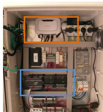
**Figure 6:** Control (in blue) and monitoring system (in orange)
