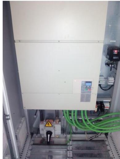
**Figure 5:** Frequency Converter
