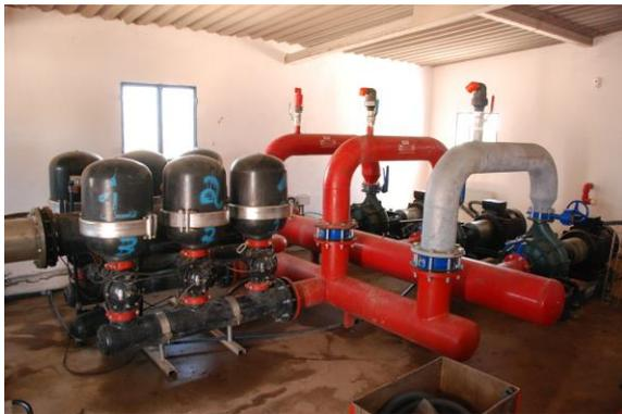
Figure 4: Set of pumps and filter bench
