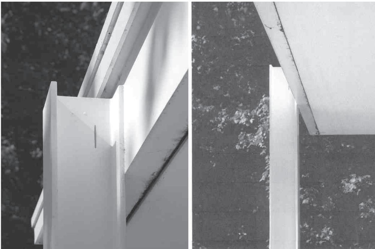
Fig. 13. The tangential union between column and beam in Farnsworth House (photo by A. Cervilla García, September 2012)
