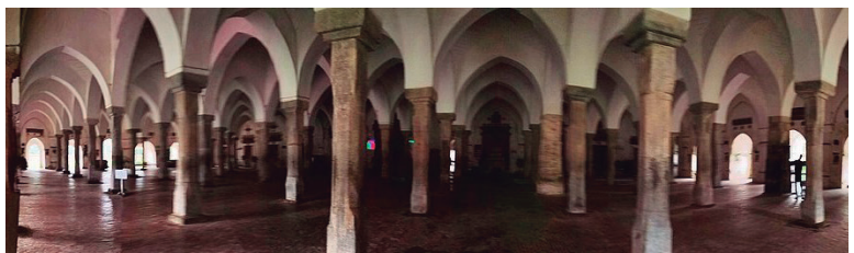
Fig. 3.257 Shatgumbad, Bagerhat (E.Hasan)
