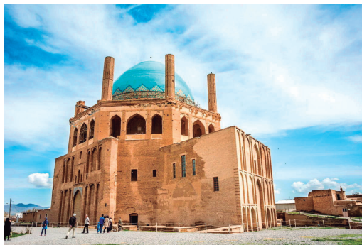
Fig. 3.229 Soltaniyeh, Zanjan (Autor)
