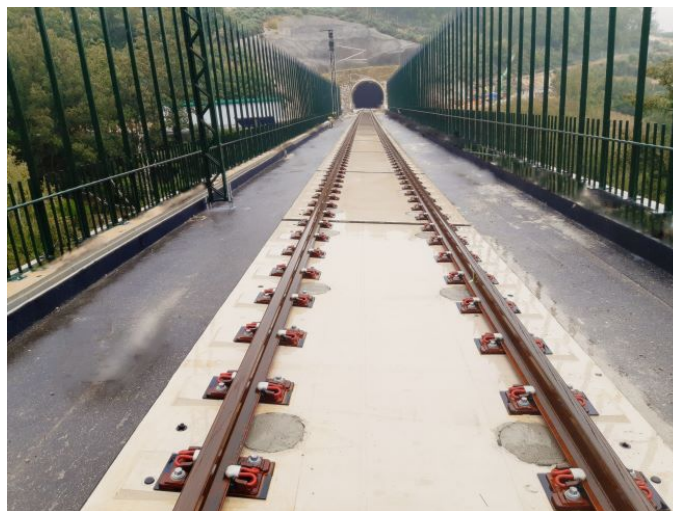
Figure 8. Prefabricated slab track system VP by AFTRAV on railway viaduct. Source: https://magazine.mafex.es/sistema-via-en-placa-vp/
