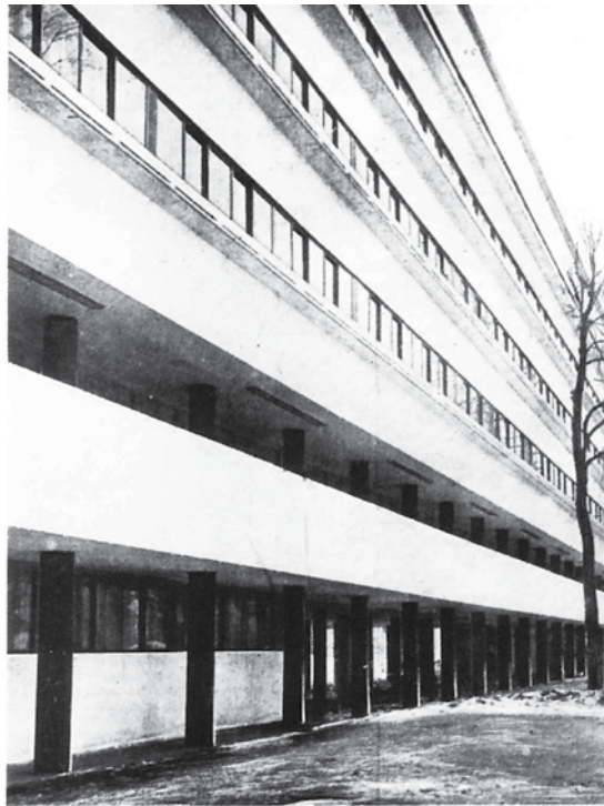
Center of building seen from the east. Ground floor, entrance to south stair. Photo taken immediately after
