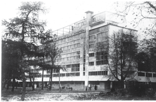
Southwest view. Top: Nikozi Mikheï's penthouse. Each apartment opens on both east and west sides of the building for light and cross-ventilation. Second and third floors with more windows. K. Ipatov
