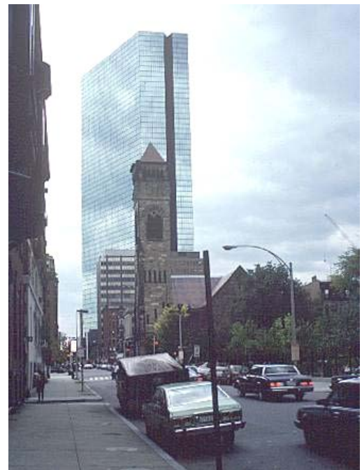
Fig. 16.- J. Hancock Building, Boston.
