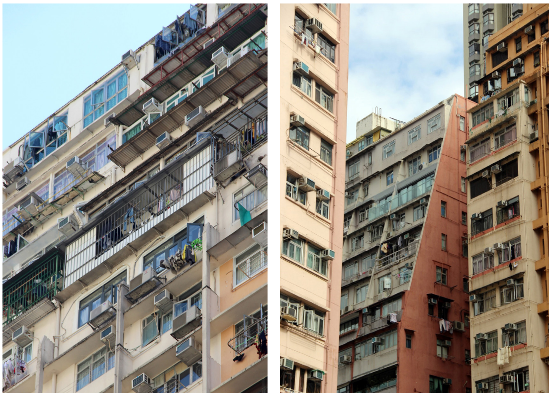
Fig. 157. 'Composite Buildings' with setbacks, 2019 and Unauthorized Building Works, Sheung Wan, Hong Kong. Source: author.
