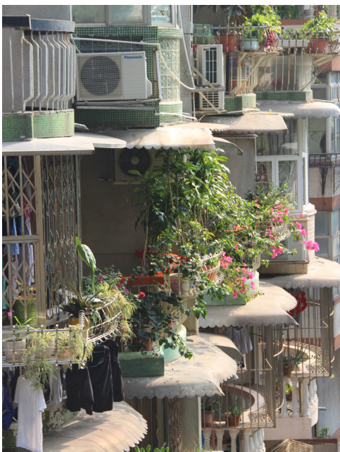
Fig. 170. (Right) Illegal cages in mid-rise apartment buildings in Bairro da Penha, Macao. New prefabricated high-rise towers are visible in the background. There, add-ons have almost dissappeared but a few can still be spot. Source: author, 2017.
