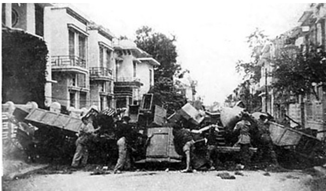
Fig. 130. Barricades in the French quarter during the First Indochina War in 1946. Source: Hanoist.
