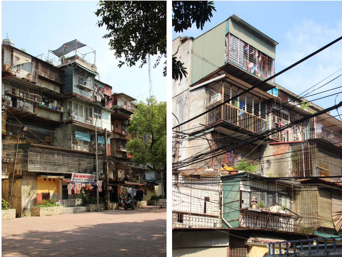
Fig. 262. Illegal apartment extensions in Thanh Xuân Bắc, Hanoi, 2019. Source: author, 2019.
