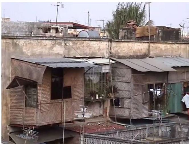
Fig. 264. Early examples of illegal housing extensions in rationalist buildings (1999), made of bamboo mats and tin sheets. Screenshots from the documentary by Nelobo Architects. 'Lines of Flight 0.1/ KTT Kim Liên (1999-2000)', 2009.
