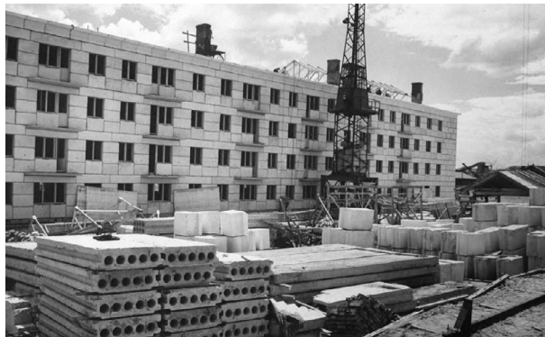
Fig. 207. Housing project for the workers of a tractor factory using prefabricated panels. Minsk, 1960. Photography by Carl Mydas. Source: Life Magazine.
