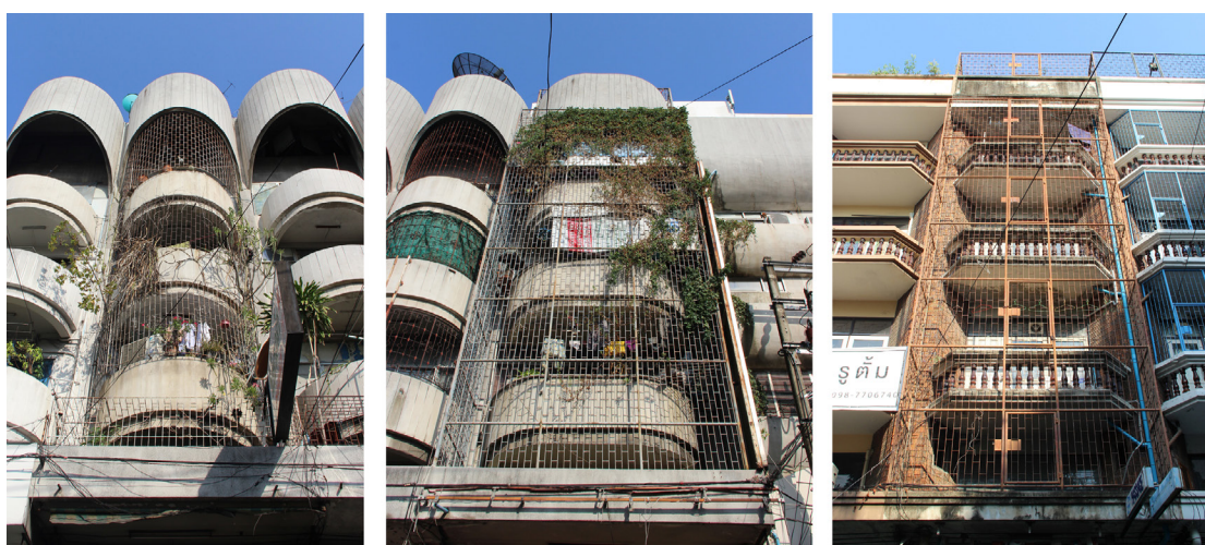
Fig. 341. Thai shophouses of reinforced concrete, known as tuekthaew , near Rama 4 expressway in Bangkok. Each unit has been covered by grilles to avoid burglaries. Source: author, 2019.
