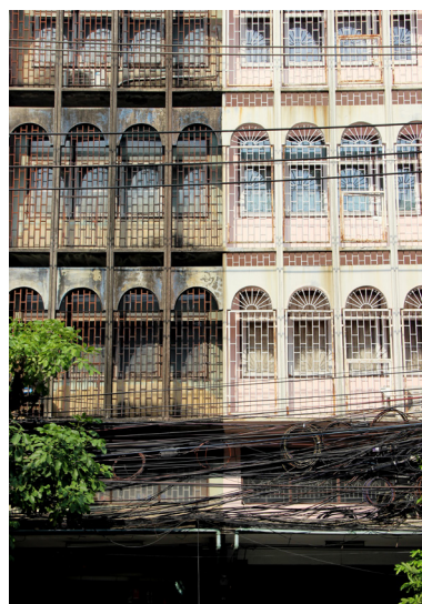
Fig. 345. Front Arched tuekthaew façades with safety enclosures in Bangkok. Source: author, 2019.
