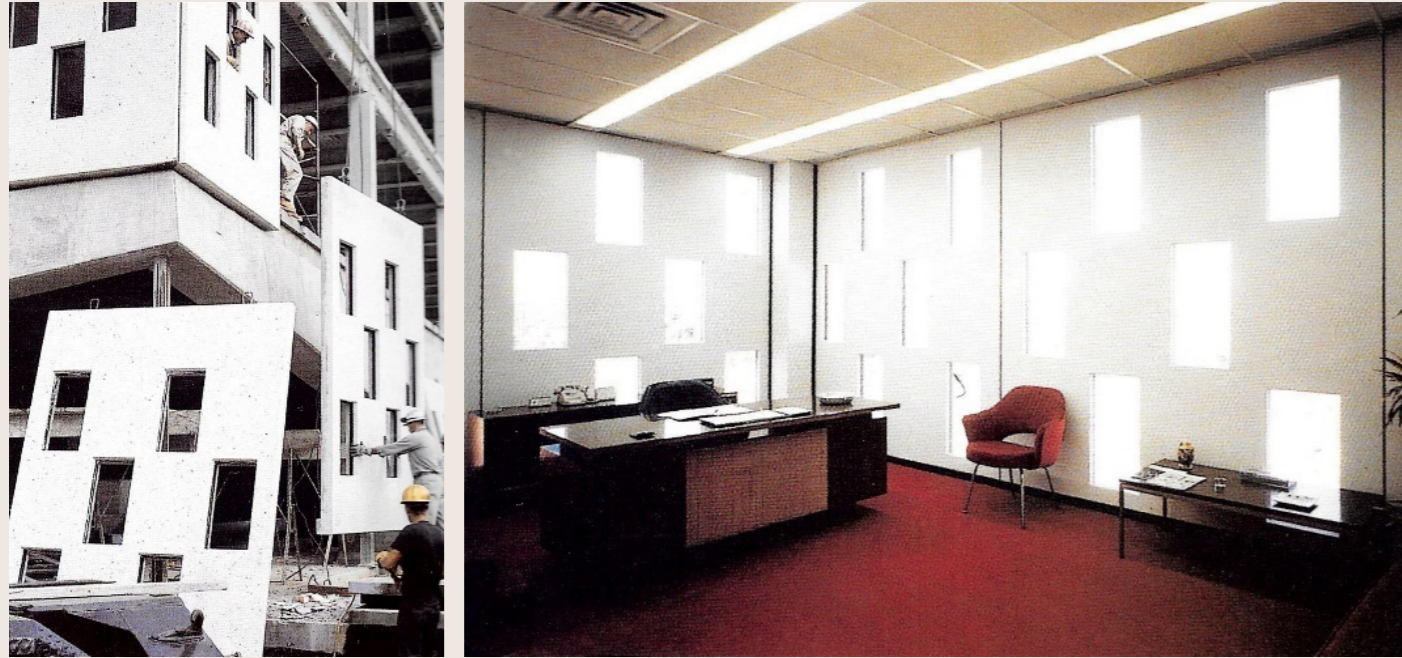
IZQUIERDA: DETALLE DE LOS PANELES PREFABRICADOS DE HORMIGÓN BLANCO DE LA CARCASA EXTERIOR. IBM AEROSPACE BUILDING. LOS ÁNGELES. CALIFORNIA. 1962. ELIOT NOYES & ASSOCIATES+QUINCY JONES+ FREDERICK EMMONS. IBM. FUENTE: BRUCE, G. (2006). ELIOT NOYES. A PIONEER OF DESIGN AND ARCHITECTURE IN THE AGE OF AMERICAN MODERNISM . LONDRES: PHAIDON PRESS, P. 178. DERECHA: IMAGEN INTERIOR DEL CONTROL DEL EXTERIOR. IBM AEROSPACE BUILDING. LOS ÁNGELES. CALIFORNIA. 1962. ELIOT NOYES & ASSOCIATES+QUINCY JONES+ FREDERICK EMMONS. IBM. FUENTE: BRUCE, G. (2006). ELIOT NOYES. A PIONEER OF DESIGN AND ARCHITECTURE IN THE AGE OF AMERICAN MODERNISM . LONDRES: PHAIDON PRESS, P. 225.
