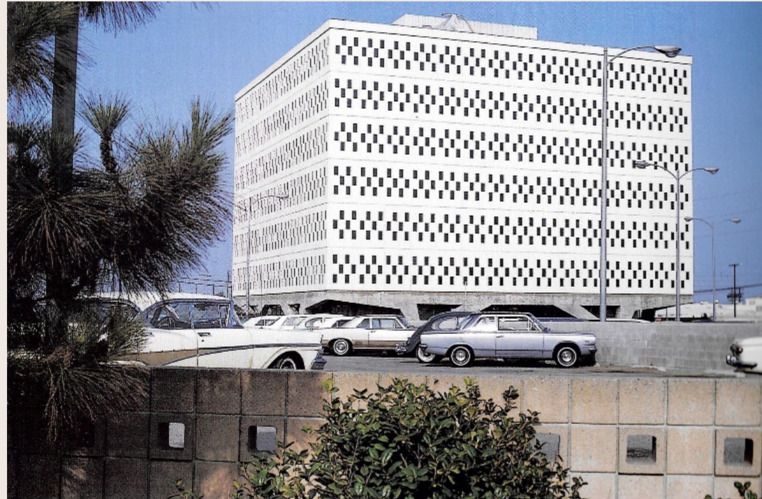
IMAGEN EXTERIOR DE LA CARCASA DEL DA IBM AEROSPACE BUILDING. LOS ÁNGELES. CALIFORNIA. 1962. ELIOT NOYES & ASSOCIATES+QUINCY JONES+ FREDERICK EMMONS. IBM. FUENTE: BRUCE, G. (2006). ELIOT NOYES. A PIONEER OF DESIGN AND ARCHITECTURE IN THE AGE OF AMERICAN MODERNISM . LONDRES: PHAIDON PRESS, P. 177.
