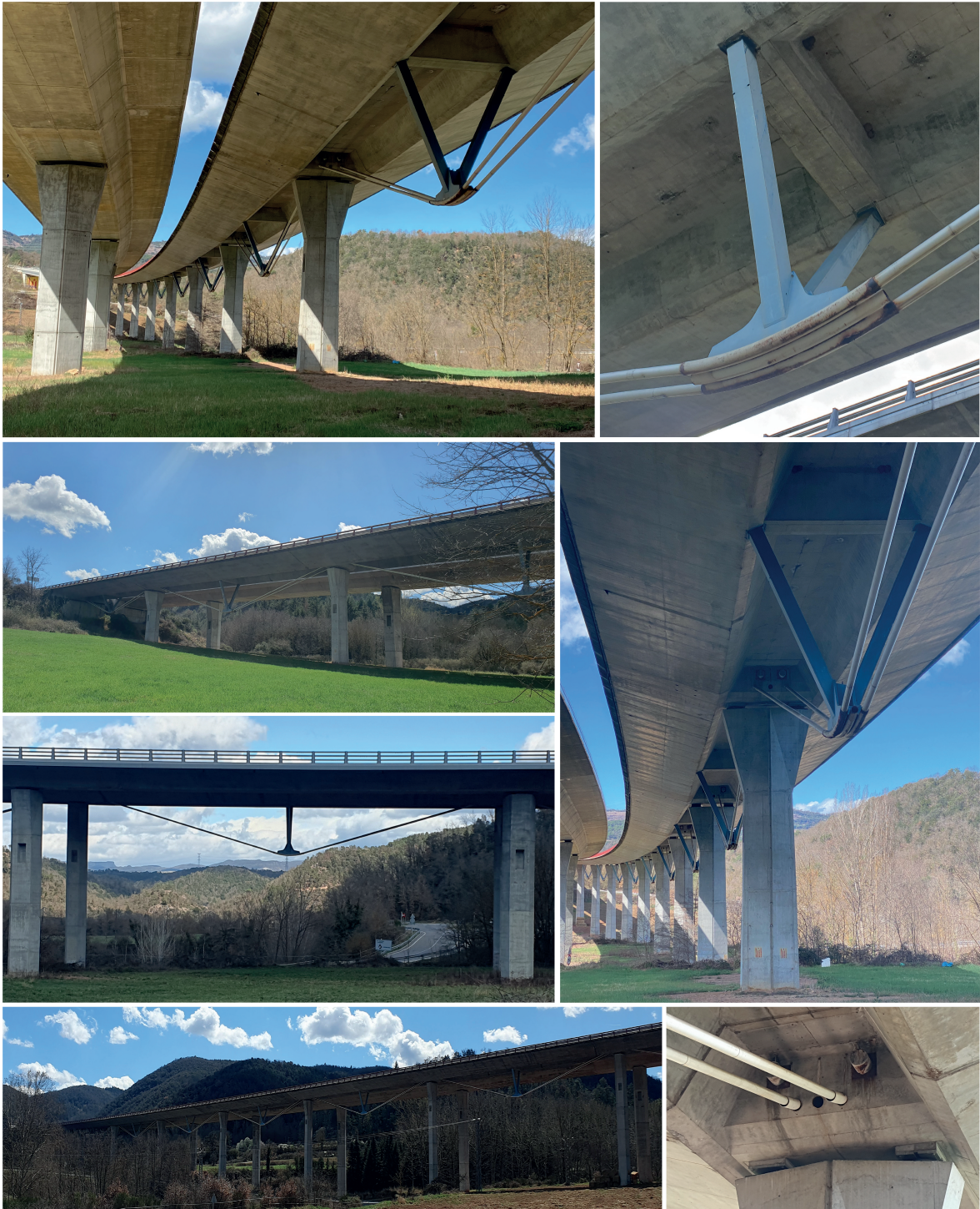
Figure 8.1: Pictures of the Osormort Viaduct, taken by the author.
