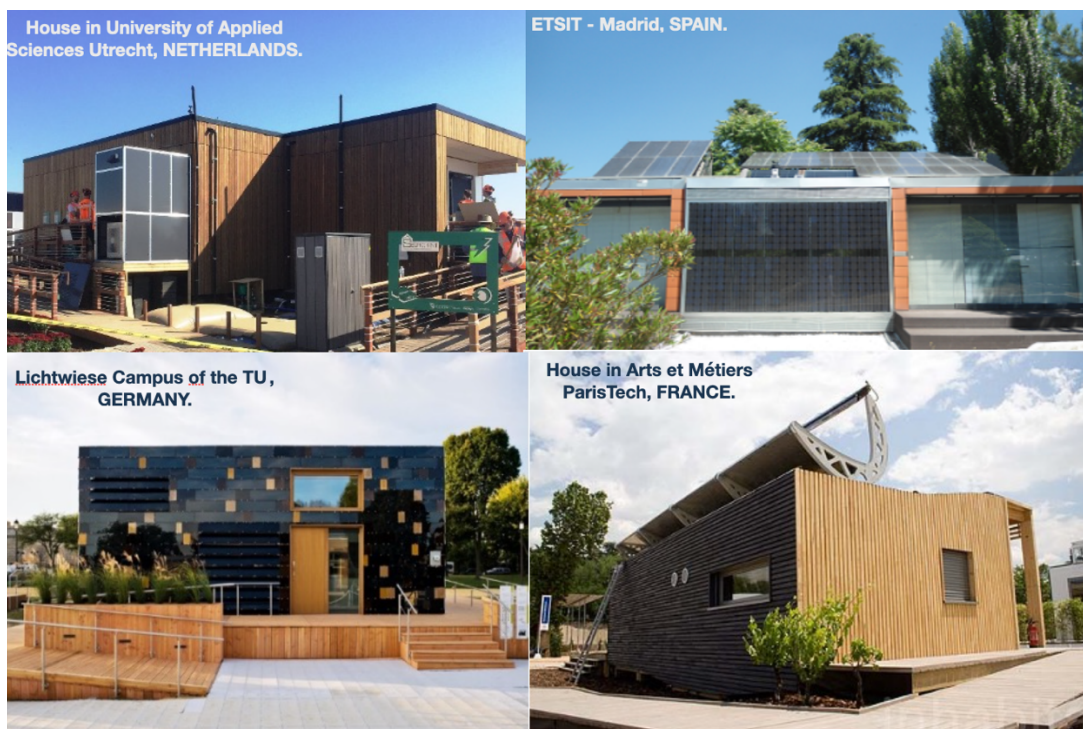
Figure 118 – Examples of European houses used as Living Labs post competition. Source: SDE Teams.
