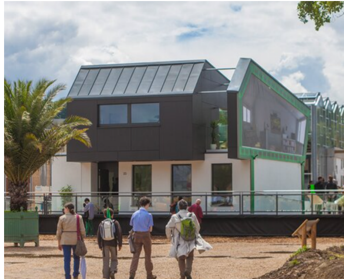
Figure 96 – On Top house. Source: SDE 2014.
