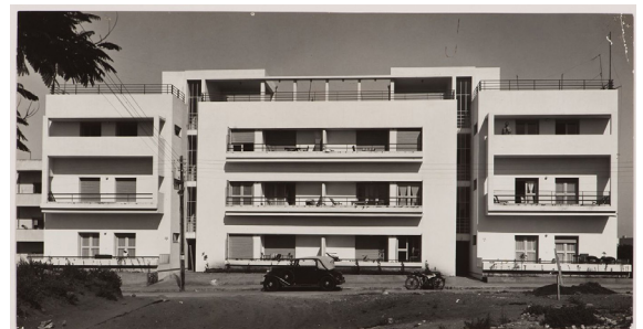
[Fig. 89] Kiryati House, Shmuel Miestechkin, 1938.
