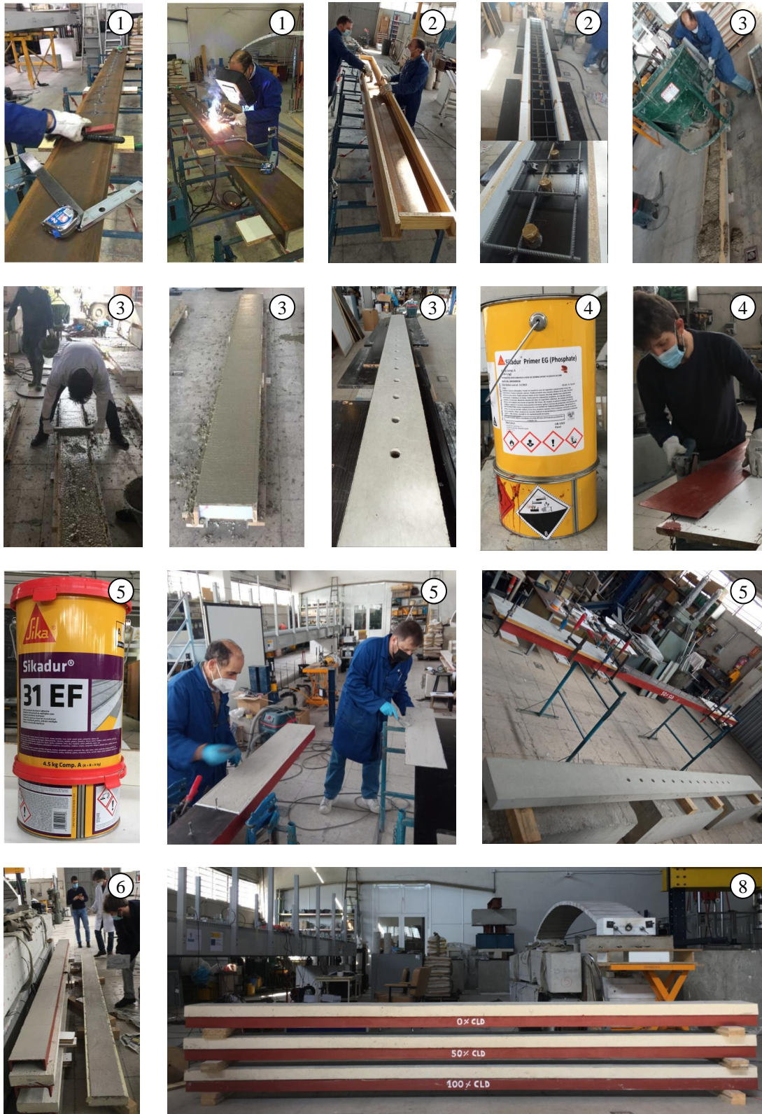
Figure 5.14: Photos related to the construction process of each RSS.
