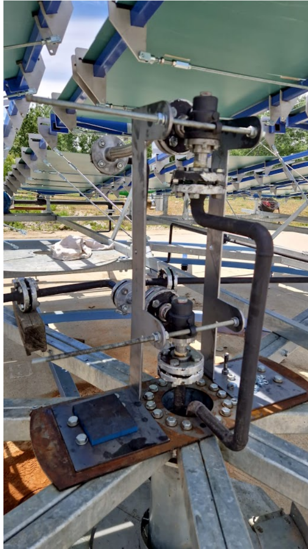
Figure 4.5: Picture of the rotatory joint assembly
