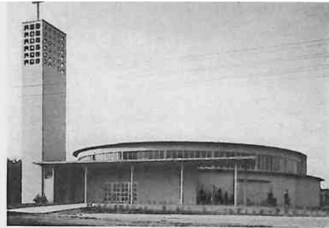
57 CHURCH OF CHRIST THE KING DAYTON AVENUE AND NORTH 117th STREET, GREENWOOD architect: PAUL THIRY 1952
