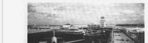
84 CLEVELAND HOPKINS AIRPORT 1956 BERA BREWERY ARCHITECTS: POCOCK, CUSHNER & ASSOCIATES This new gateway to Cleveland is distinctive for its efficient circulation pattern. Concourses radiate from the central building to the landing field; the depressed drive around the main building, used by service vehicles, segregates pedestrians and carries handsome non-bearing walls and partitions provide flexibility. The entrance features metal sculpture.
