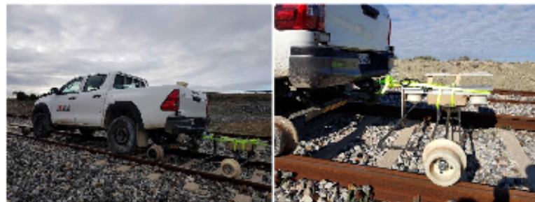
FIGURE 21 Assembling of the equipment for developing the test 3 on railway track 2.
