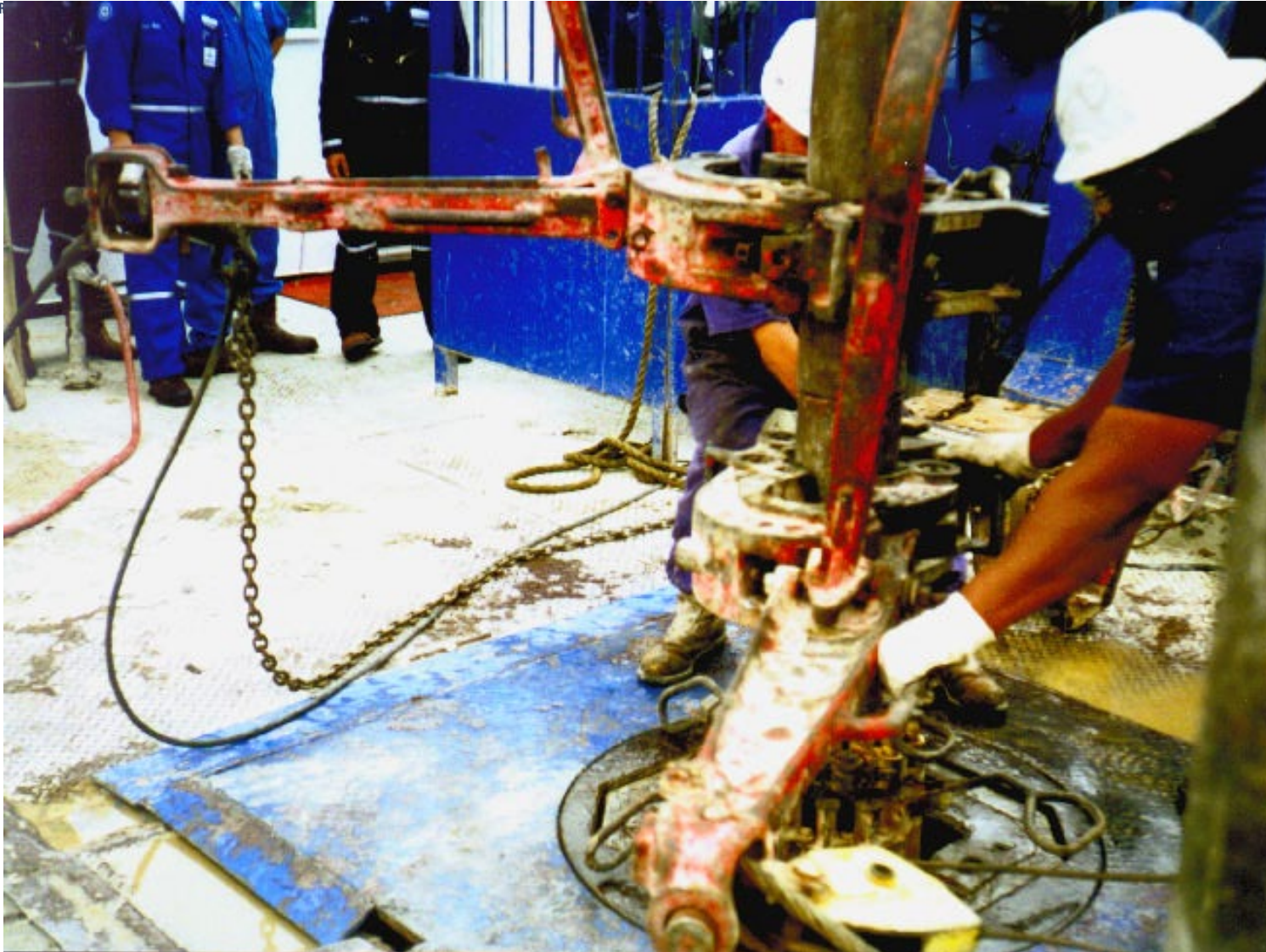
Applying the torque to the joint
