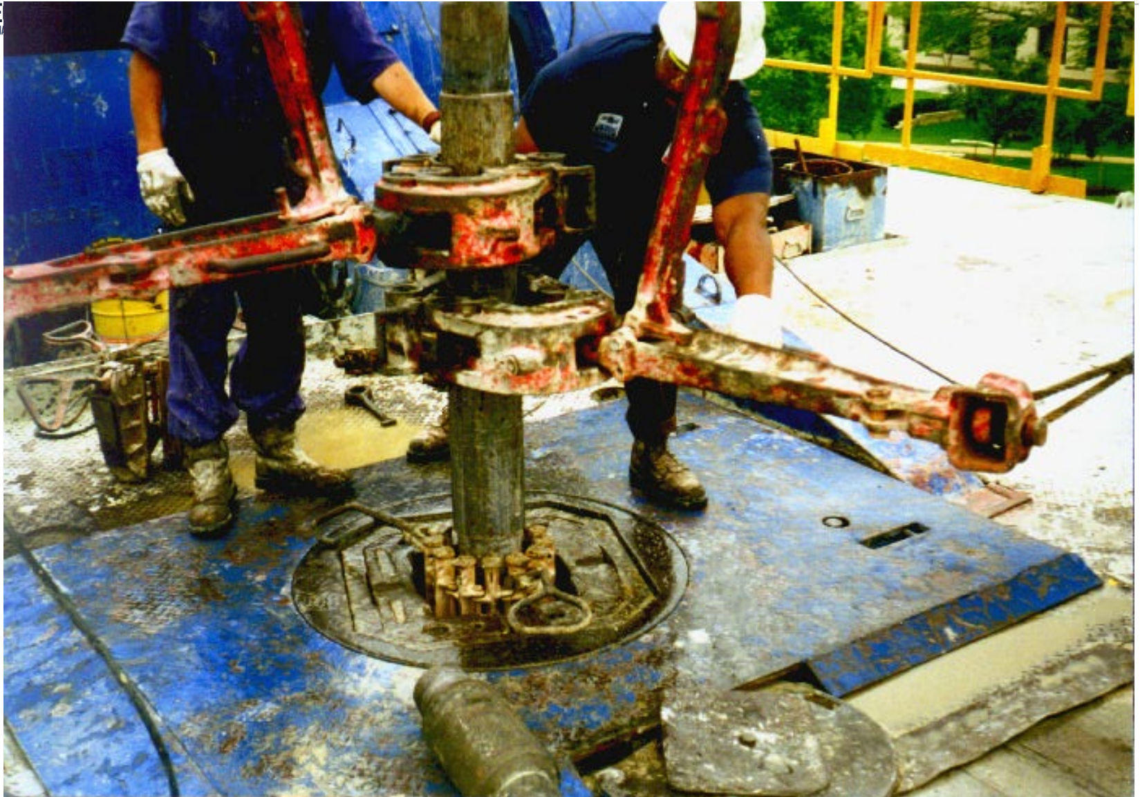
Applying the torque to the joint
