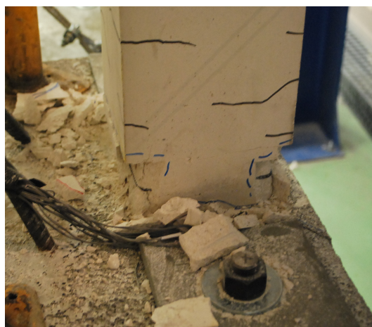
Figure 4: Specimen BS. Final state of exterior column C1
