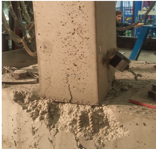
Figure 5: Specimen BS1. Final state of exterior column C1
