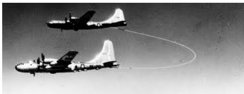
Figure 1.2: Grappled-Line Looped-Hose Air-to-Air Refueling in 1935.
