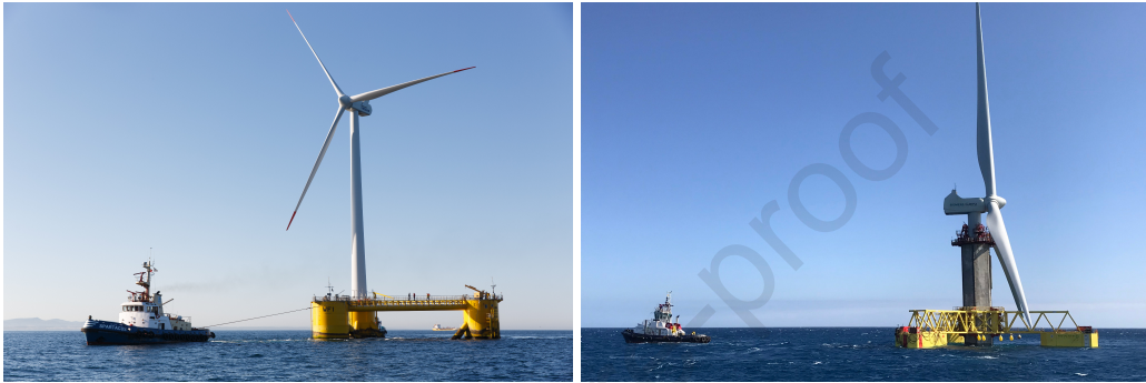
Figure 1: Towing maneuver of WindFloat unit, left (credits to Recharge, Oslo, Norway) and ESTEYCO's ELICAN, right (credits to ESTEYCO).
