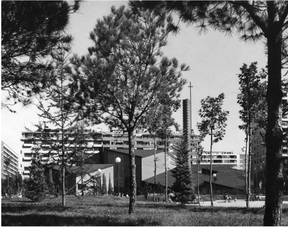
7.6 Exterior view of the San Fernando parish complex (1970) (Luis Cubillo de Arteaga, architect). [Courtesy of Cubillo de Arteaga Legacy (LCA.Foo7), Madrid, ASHCOAM]
