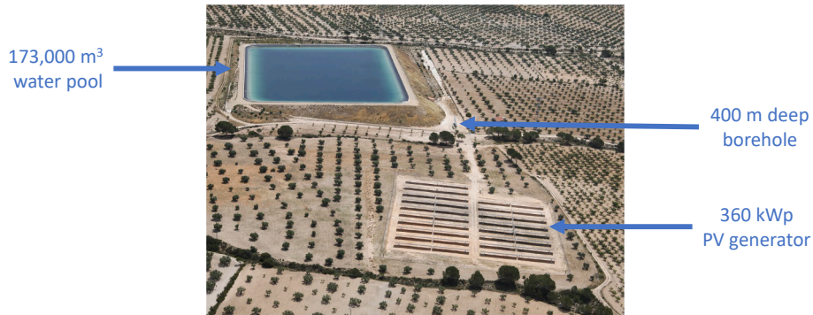
Fig. 3. PV irrigation system in Villena.
