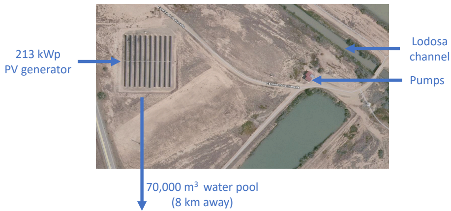
Fig. 6. Aerial view of PV irrigation system in Aldeanueva.
