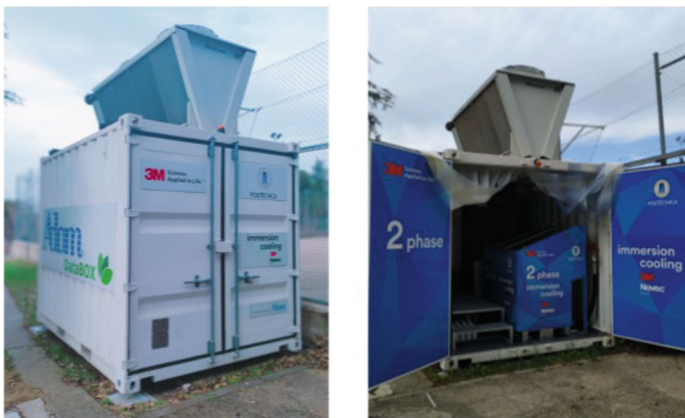
FIGURE 8 Two-phase immersion cooling EDC prototype.
