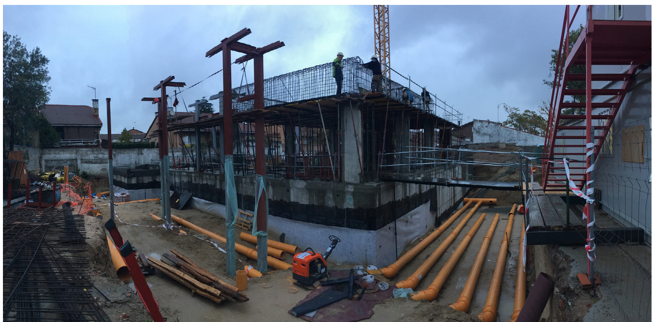
Figure 6. Construction of the BRAINS school. Installation of the Canadian wells.
