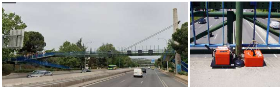
(a) South view for the A6 highway.
