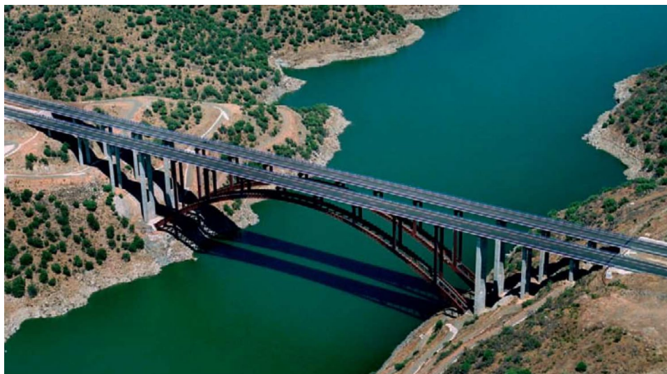
Fig. 12 Viaduct “The Arches of Alconétar”; general aerial view
