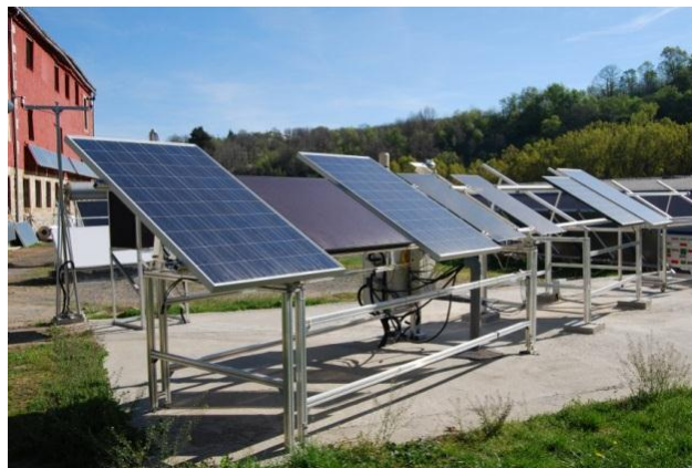
Figure 3-4: Modules placed in the test bench. The UMG one is the first from the left and the standard the third.
