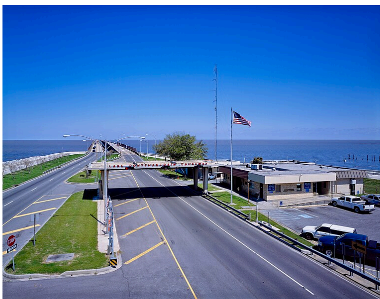
Figure 3. South Lake Pontchartrain Causeway Toll Plaza, Metairie. Source: Historic American Engineering Survey photo via Library of Congress website at https://www.loc.gov/re-source/hhh.la0640.photos/?sp=2&st=image
