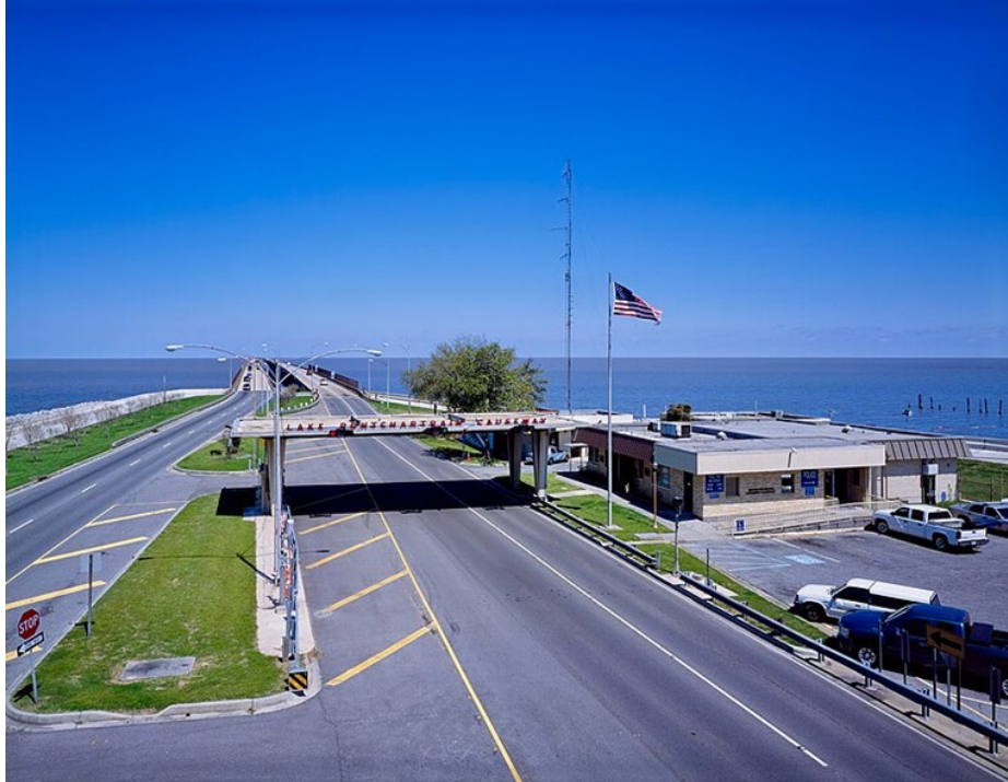
Figura 2.43: Plaza de peaje del sur de la calzada del lago Pontchartrain, Metairie. Fuente: Historic American Engineering Survey photo via Library of Congress website at https://www.loc.gov/resource/hhh.la0640.photos/?sp=2&st=image
