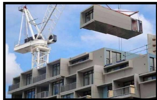
Figure 5: prefabricated parts (21)
