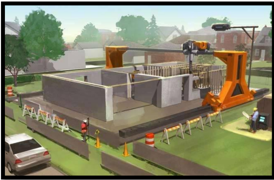
Figure 1. Construction with 3D printers (Source : www.edelplast.com/3Dprinter )
