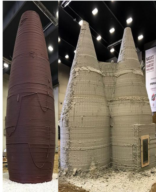
Figure 13: 3D-Printed Extraterrestrial Habitats (66)
