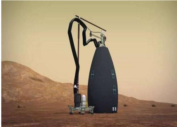
Figure 4. construction of the settlement by 3D printer (Madeleine, 2022)
