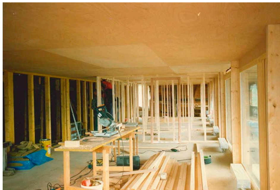
Figure 16. Walenstadtberg Housing under construction. Timber frame construction on the first floor. Material provided by Gody Kühnis.
