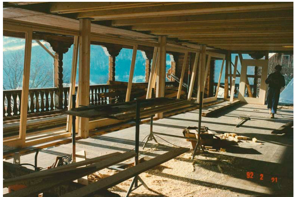
Figure 10. Walenstadtberg Housing under construction. The placing of the wooden windows between columns of what we have called the glazed loggia. Material provided by Gody Kühnis.
