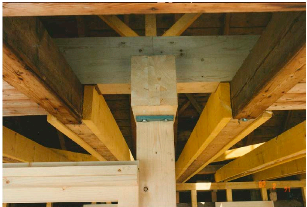
Figure 18. Walenstadtberg Housing. The reinforcement of the upper timber floor slab and fixing of the new pillars on the southwest façade. Material provided by Gody Kühnis.
