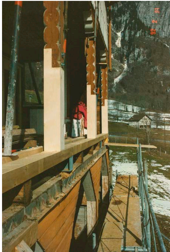
Figure 17. Walenstadtberg Housing. The repair of the pillars of the veranda by replacing the damaged parts. Material provided by Gody Kühnis.
