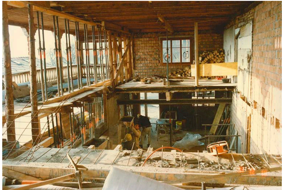
Figure 9. Walenstadtberg Housing under construction. Note the brick shell on the southwest and northwest façades of the ground and first floors. The new timber frame construction will be housed inside. Material provided by Gody Kühnis.
