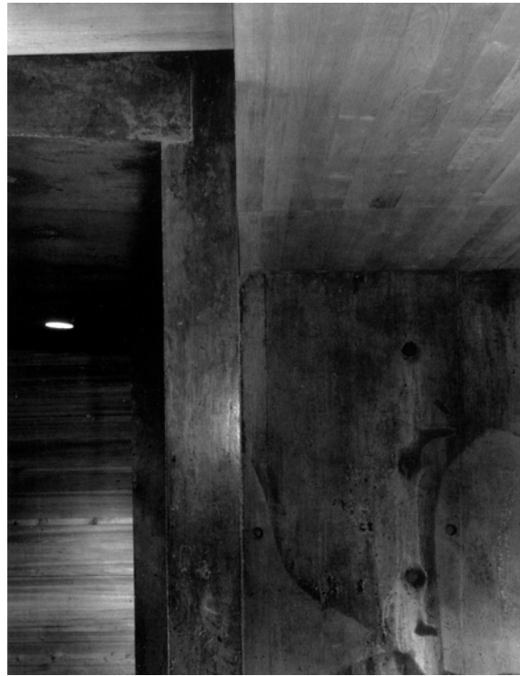
Figure 34. Gugalun House black beast upper corner of the black concrete slab-wall between the kitchen ( left ) and the dining room ( right ). Orthos Logos.
