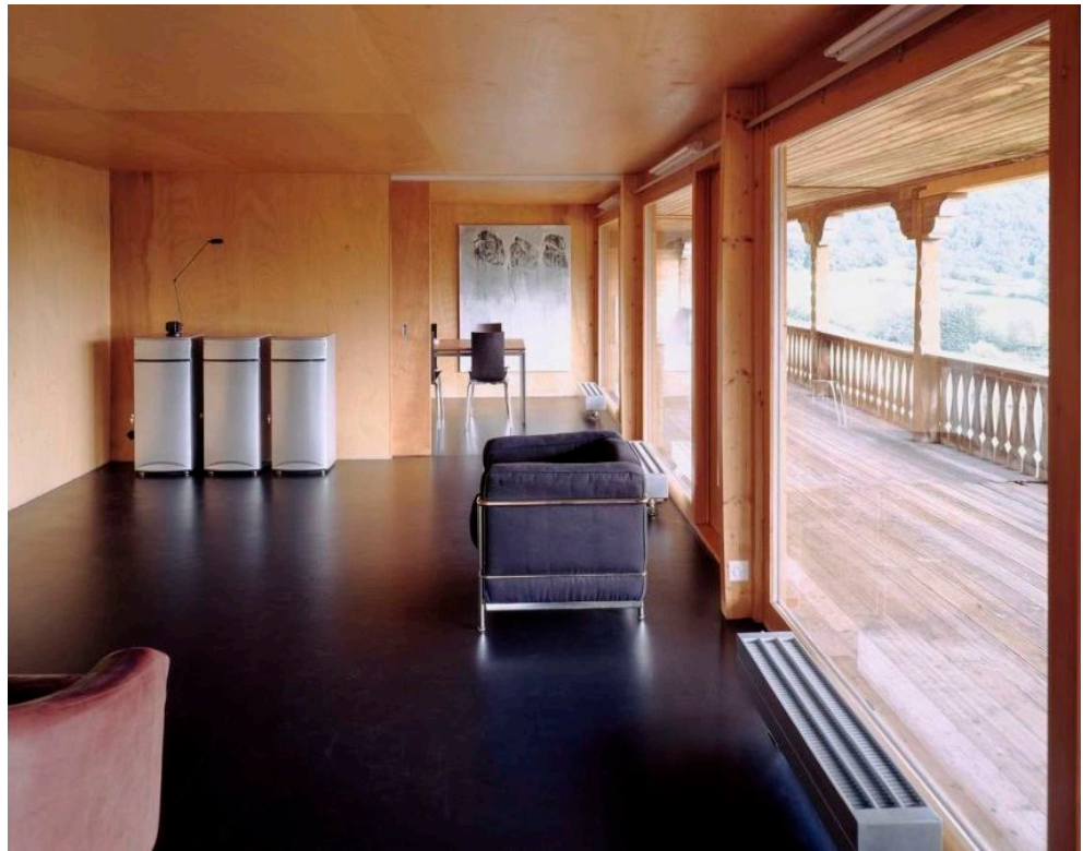
Figure 19. Walenstadtberg Housing. The first floor finished with wooden cladding and linoleum floor. Note the entasis of the free-standing pillars of the façade [12].
