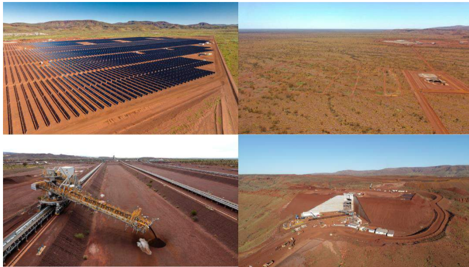
Fig. 9 Gudai-Darri Mine in Australia
