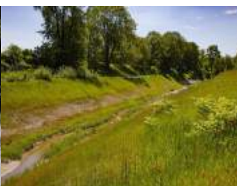
Fig. 15 Resser Bach after restoration
