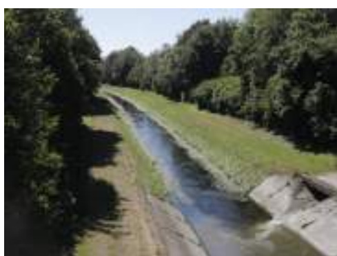
Fig. 14 Nettebach after restoration
