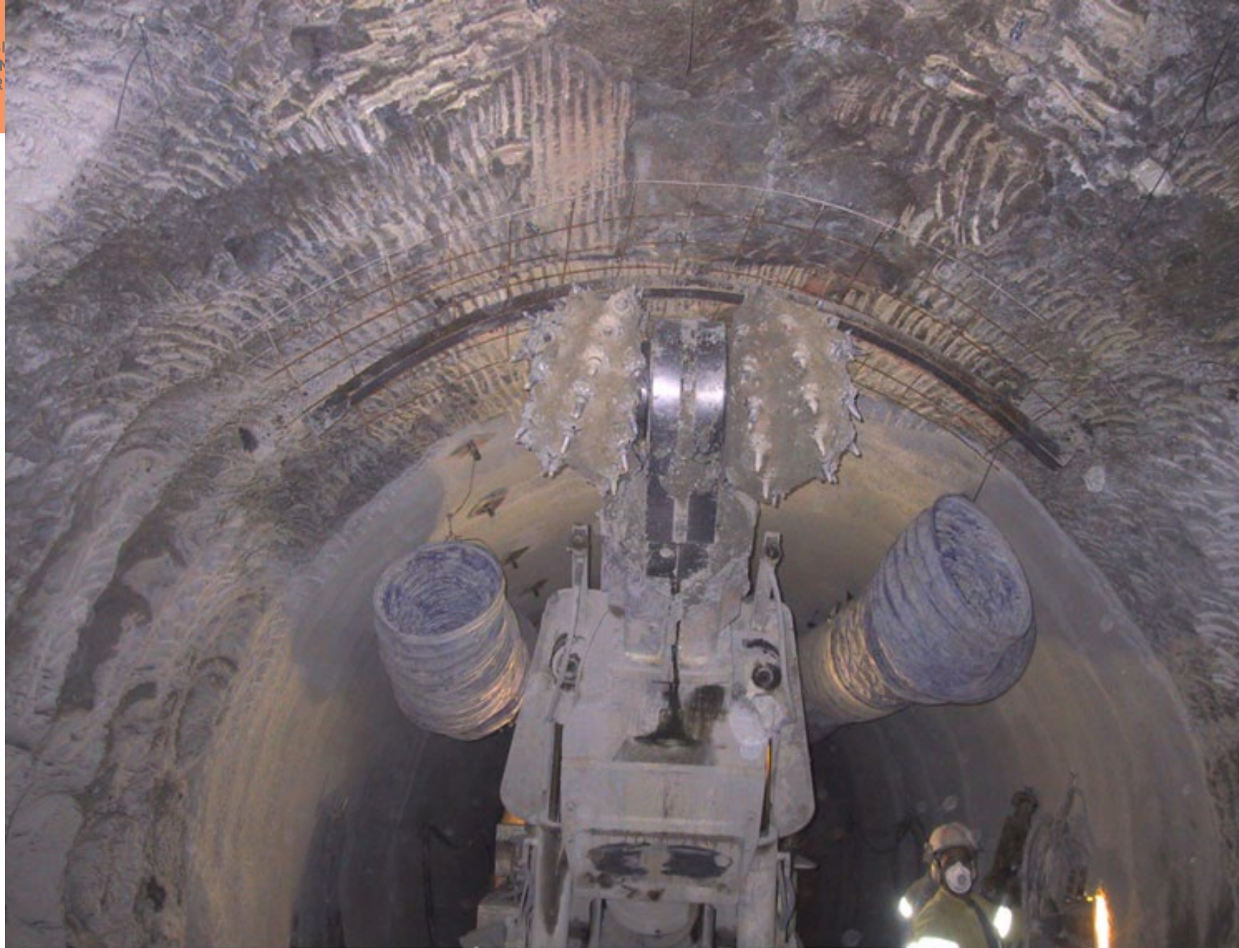
CNGS - Proton beam tunnel excavation by roadheader - November 20, 2001 - CERN ST-CE
