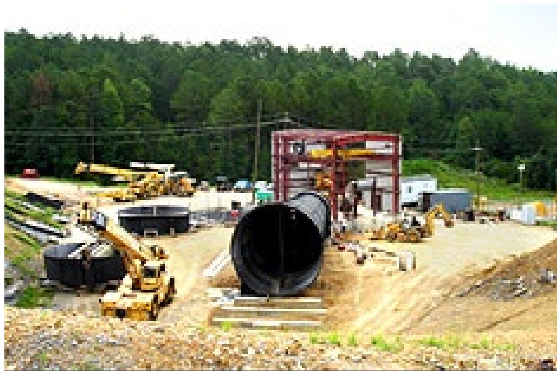
Construction of Fan Building.
