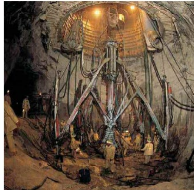
A typical pneumatic shaft jumbo
