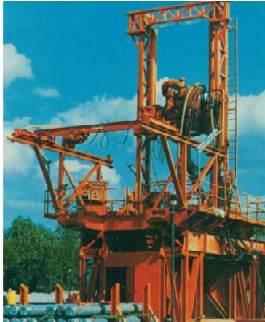
Hughes large-diameter drill rig
