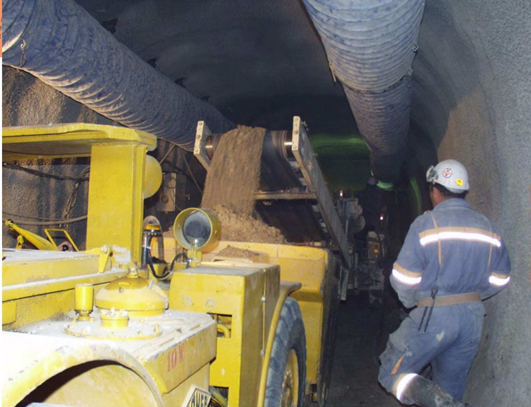
CNGS - Roadheader proton beam tunnel - August 01, 2001 - CERN ST-CE
