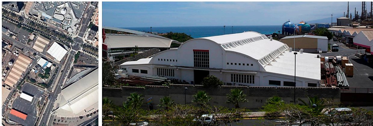
Figure 8. The machinery warehouse of the refinery, by architect José Blasco Robles (c.1957), catalogued in DOCOMOMO, is notable for its constructive and plastic values. The structure is formed by a combination of longitudinally directed warehouses, topped by others with a transverse direction. However, it was shortened by one-third of its total length due to the construction of the avenue next to it. It was previously protected as a cultural heritage site. Assembly by JDLA.
