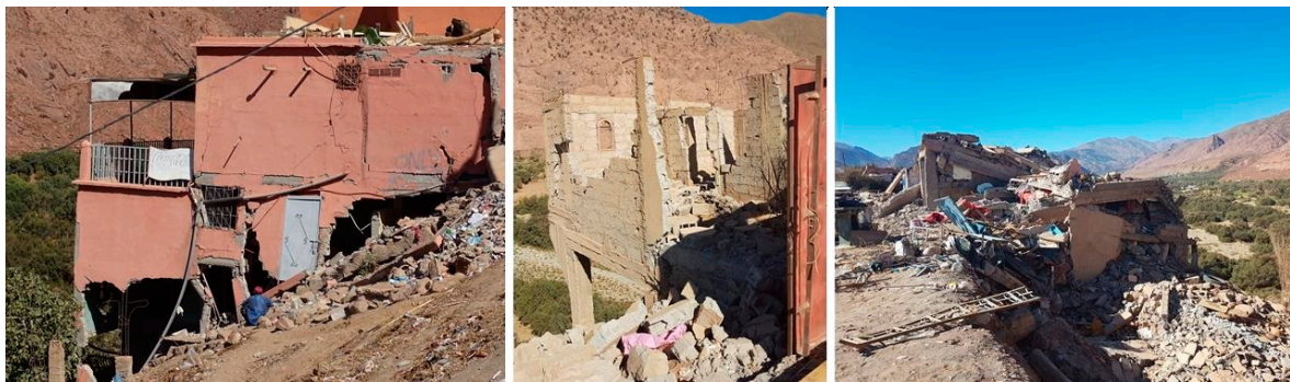
Figure 28. Buildings located on slopes and presenting very different column lengths (Talat N'Yaaqoud).
