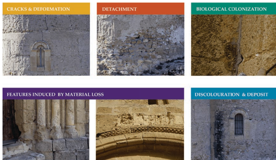
Figure 5. Stone weathering following ICOMOS terminology.
